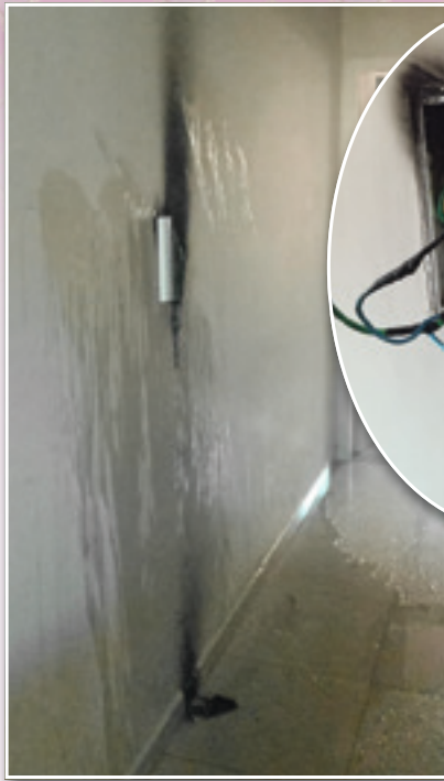
The fuse box after the fire
